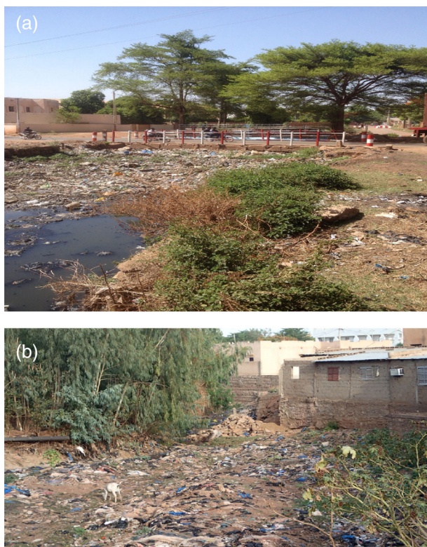
FIGURE 9 (a) Example of a collector clogged by litter at Cité Niger, Bamako (12.642591, -7.976238). Photo taken on 20 May 2017. Copyright F. Cazenave. (b) Example of a house built in the inundation bed in Bamako (12.681323, -7.922695). Photo taken on 28 April 2016. Copyright F. Cazenave.
