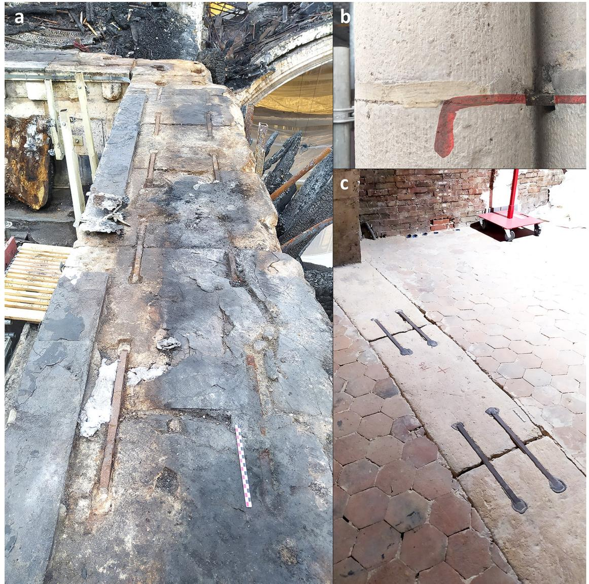
**Fig 1. Iron armatures in Notre-Dame.** a. Iron staples of the top walls (southern nave looking on the angle of the southern transept). b. Iron staples inside the monolithic columns of the nave (view of the staple in red). c. Iron staples in the tribunes of the choir (staples n° 121 to 124).
