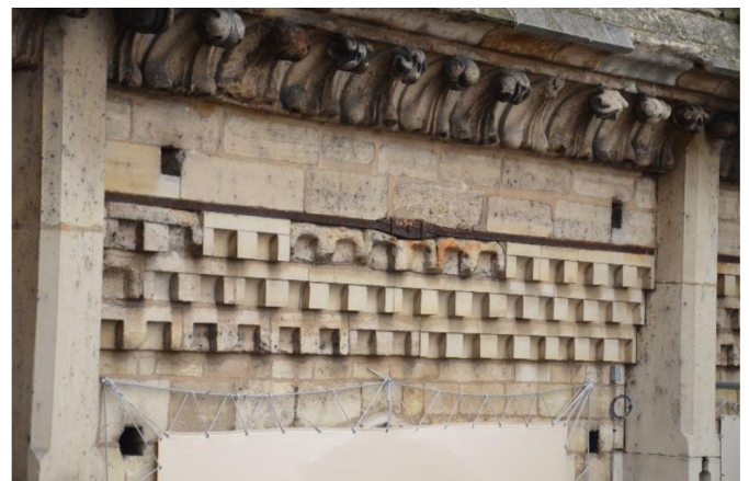
Fig 3. View of the checked cornice of the choir with its series of staples drawn by Viollet-le-Duc (left) [19 tome 2, p. 400] and today, with the chains implemented by Lassus (right).
