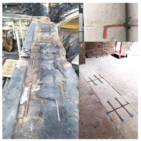
**Fig 1. Iron armatures in Notre-Dame.** a. Iron staples of the top walls (southern nave looking on the angle of the southern transept). b. Iron staples inside the monolithic columns of the nave (view of the staple in red). c. Iron staples in the tribunes of the choir (staples  $n^{\circ}$  121 to 124).
