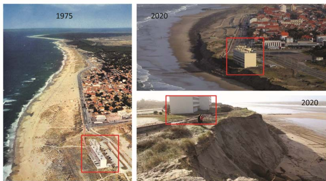
Fig. 1. "Le Signal", building in Soulac-sur-Mer (Gironde): evolution of coastal erosion (source: Région Aquitaine-La Dépêche-Philippe Clairay).
