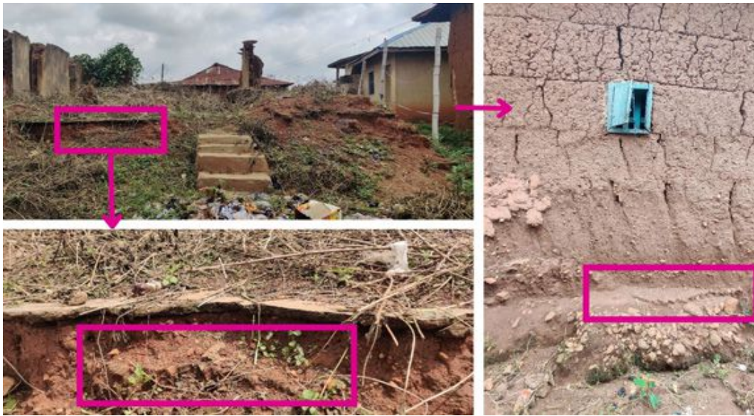
FIGURE 1. General view of the Lújùmò Compound, Ilé-Ifẹ̀. Left: view of the ruins of the house with the pavements visible below the modern cement-floor level; right: neighboring rammed-earth house with pavements appearing at the foundation level. (Photos courtesy of Léa Roth, 2021.)
