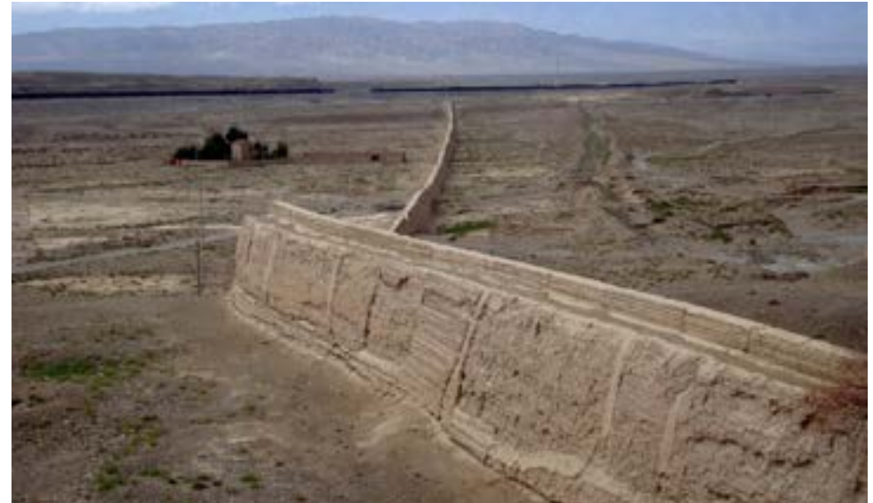
Portions of the Great Wall built with earth © Gwydion Williams (Flickr, creative commons)
