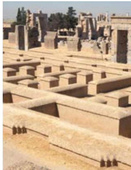
Detail, restored earth walls © David Gandreau, CRAterre
