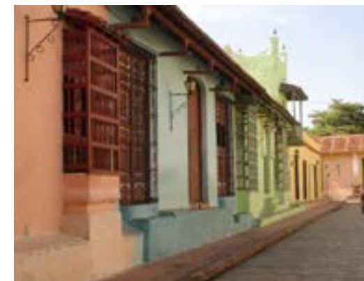
Facades, 18th and 19th centuries in wattle and daub © OHC Camagüey
