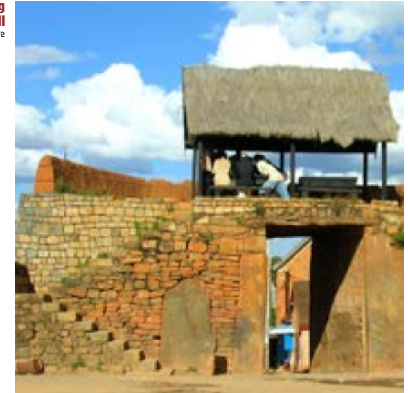
Earth and stone fortified gate, giving access to the sacred hill © Sébastien Moriset, CRAterre
