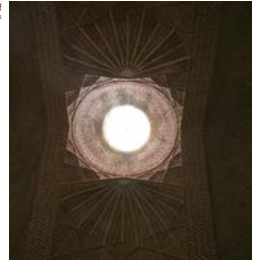
Detail of vaulted roof © Mohammad Tajik
