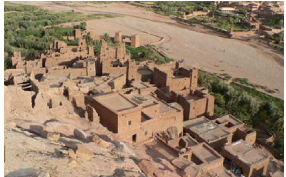
The site, the oued and the new town as seen from the hill © Sébastien Moriset, CRAterre
