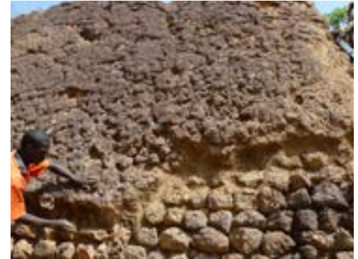
Conservation of earth plaster covering the laterite blocks © David Gandreau, CRAterre
