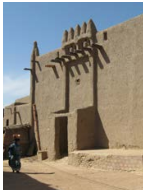
Earten house in Djenné © Thierry Joffroy, CRAterre
