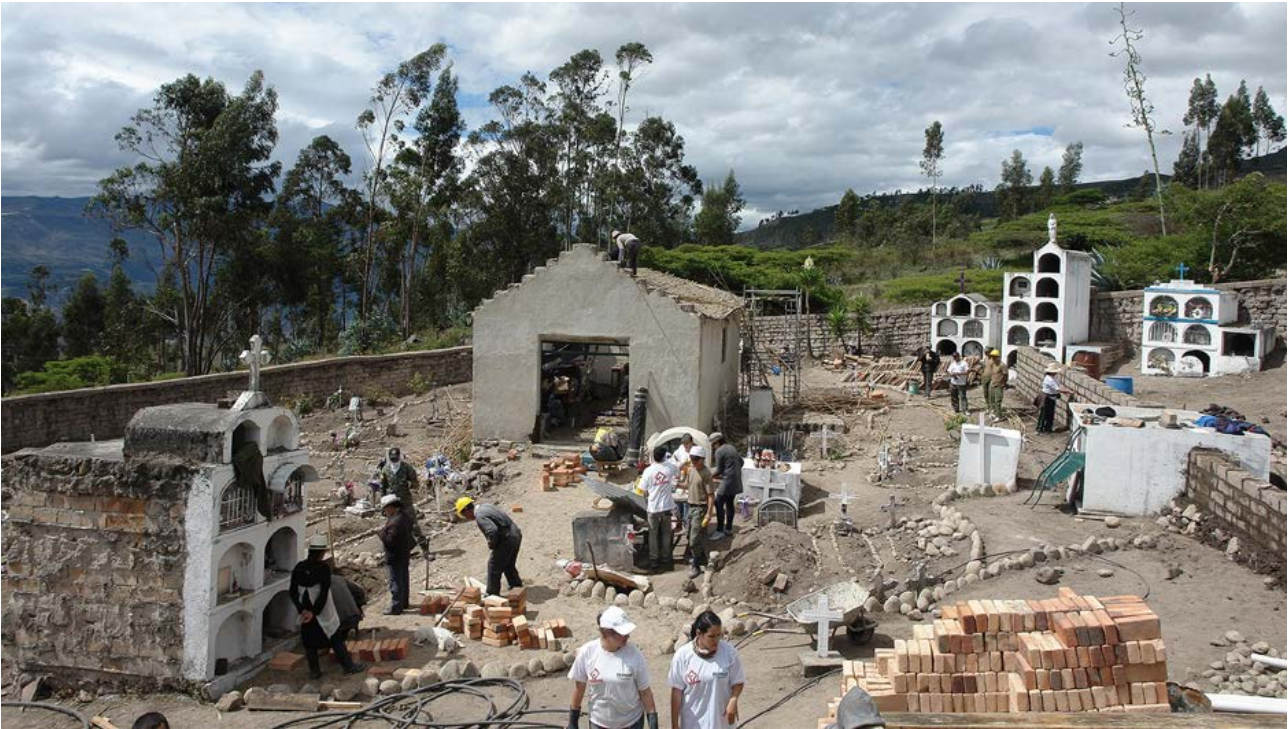
Fig. 4: Intervention processes of the heritage cemetery of Susudel. Source: CPM Project
