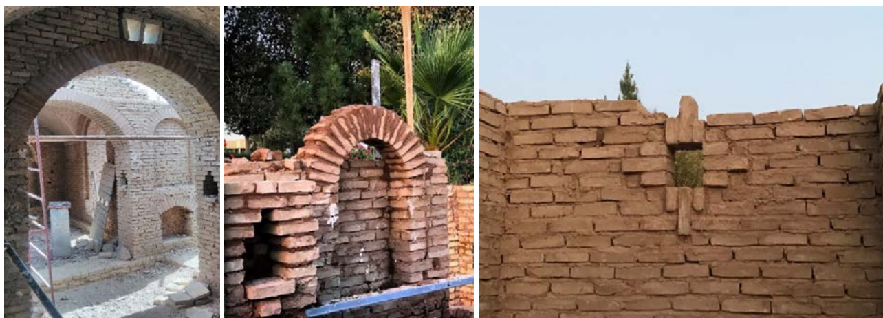
Pictures 1, 2 and 3. Innovative on site details by "Arman"
