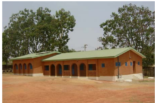
Fig.1: The Centre for French Teaching and Documentation(CFTD), Jos one of the demonstration buildings constructed by CECTech using CEB
