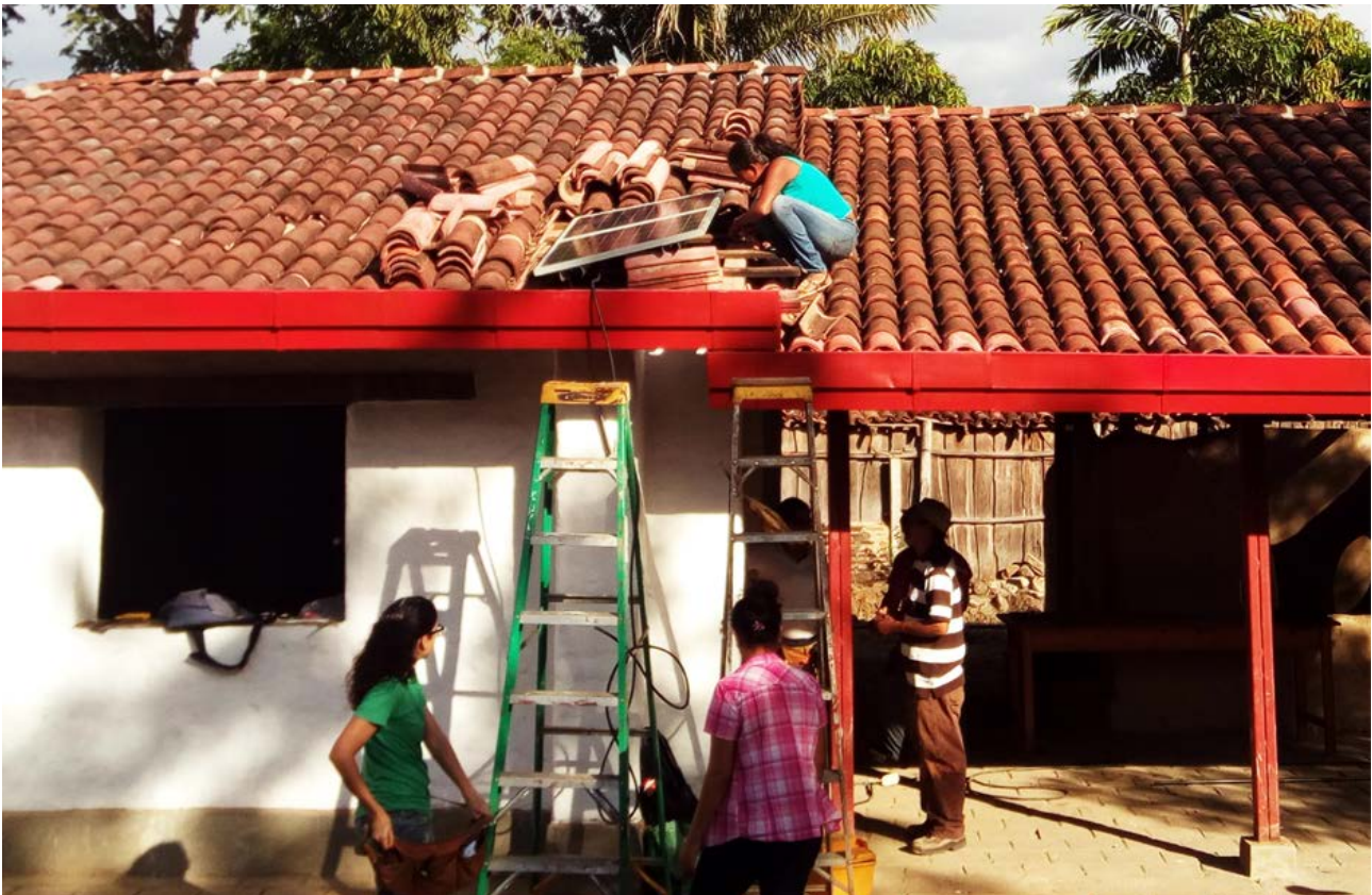
Fig.5: Installation and maintenance of solar photovoltaic energy systems course, 2016, AMCC
