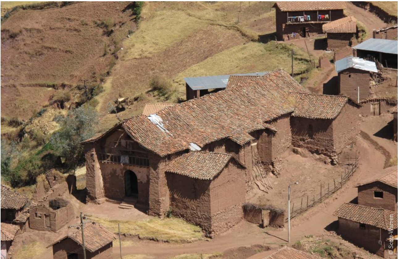
Fig. 1 : Church of Kuñotambo before intervention
