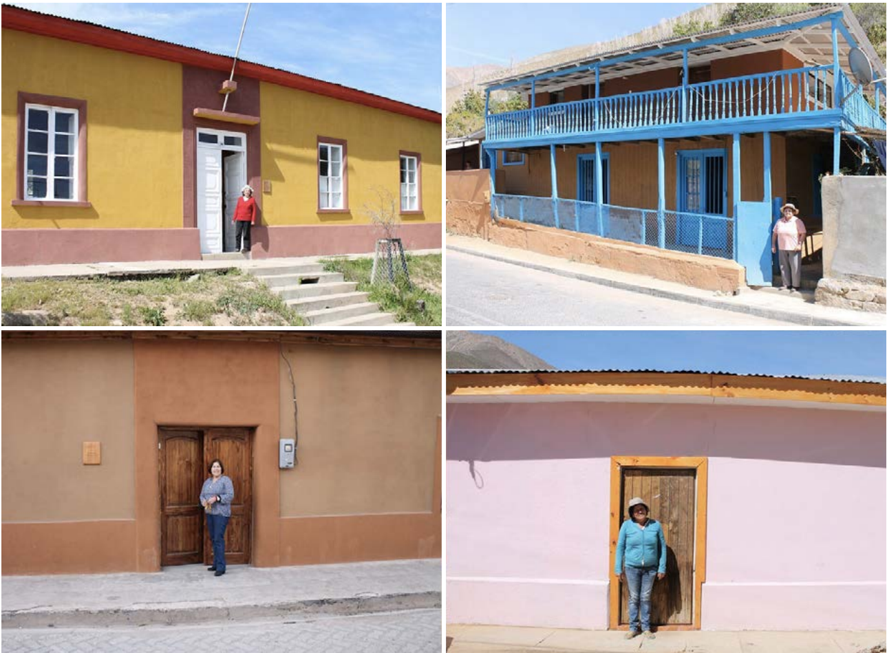
Fig.3: Houses repaired with the program of Heritage Reconstruction of the Housing Ministry (© Solange Miranda Coletti)
