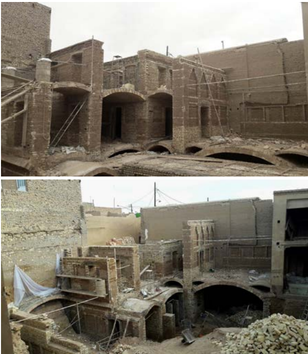
Fig 4, 5. New building made of mud bricks using traditional techniques, source: ICHHTO archives
