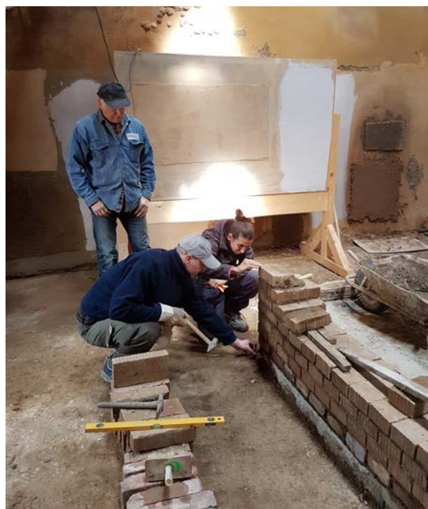
Fig.1: "Learn Earth" course B1+B2 Earthen Brick Masonry in 2017 Fig.2: Professional qualification "Contractor of clay constructions" examinations pursuant to Act No. 179/2006 Coll., in 2017
