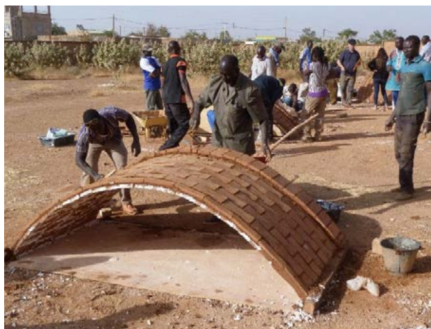
Fig.5: Workshops for the construction of tile vaults with CEBs (Burkina Faso 2018)
