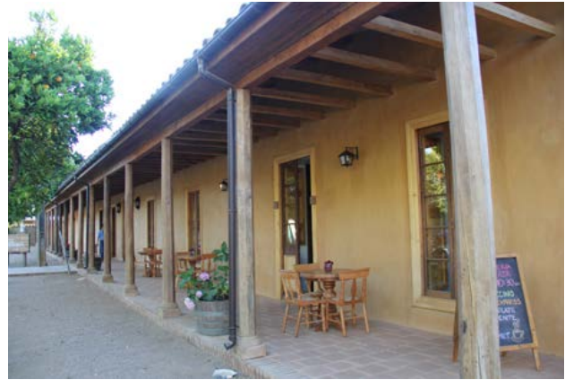
Fig. 1b: Repaired houses in the historic centre of Vichuquén
