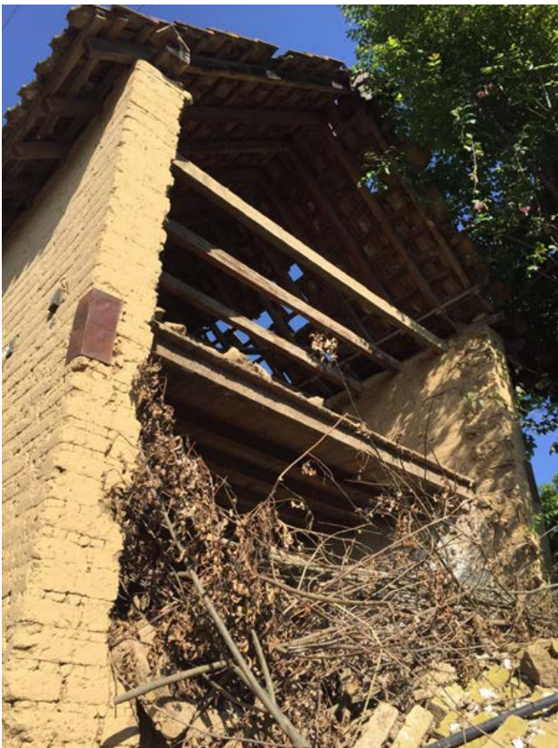
Fig 5: The "braces" or tensors confine the longitudinal walls. Ocuituco, Morelos
