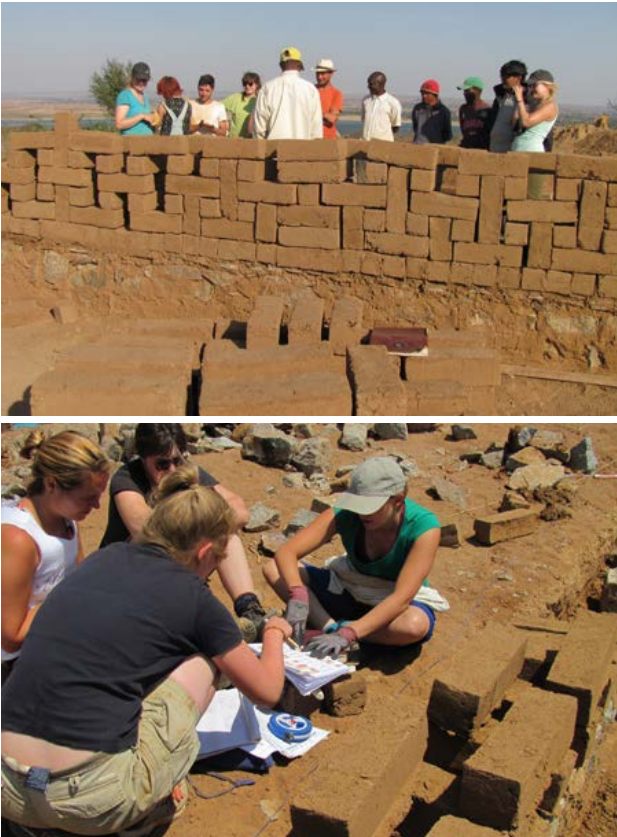
Fig.4&5: International participants of the Singida Earth House Workshop in Tanzania 2016, checking variations of masonry layers before final erection of walls (above) and checking draft and built walls
