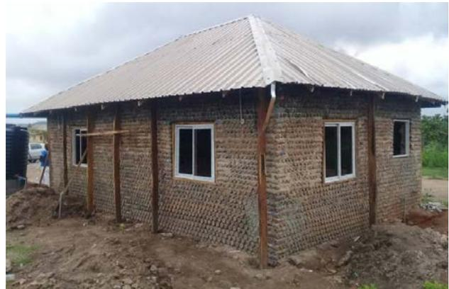
Fig.5: The DMU-IESD's low impact housing using earth and recycled plastic bottles, Mpape (Païpe), Abuja-Nigeria
