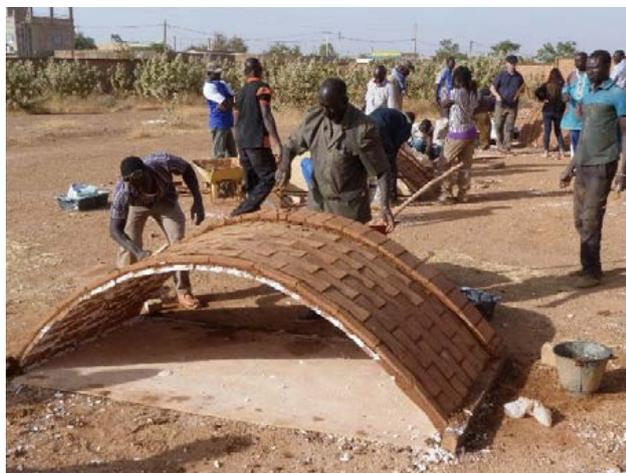
Fig.5: Workshops for the construction of tile vaults with CEBs (Burkina Faso 2018)
