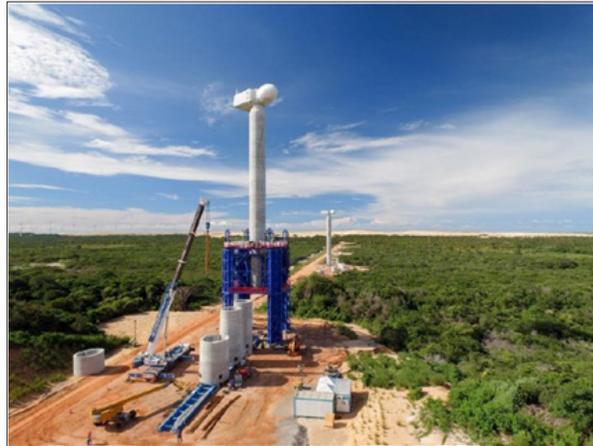
**Figure 1:** Tower erection (EOLIFT system).
