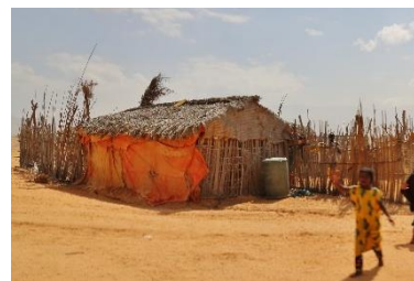
Baraako without plaster and with palm leaves roof in Puntland – CC Heimo Liendl
