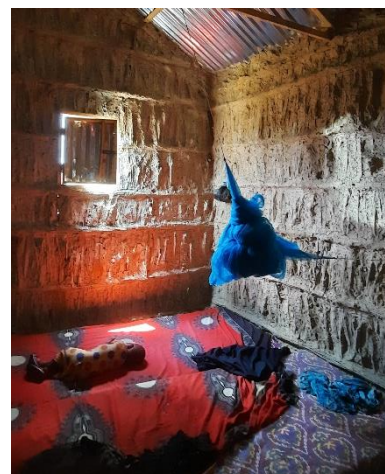
Earth construction provides comfort thanks to its thermal inertia and to its capacity for moisture regulation. Baraako and mundul also offer ventilation thanks to micro cracks in earth plaster. Baidoa, South West State – CC Enrique Sevillano Gutiérrez, CRAterre
