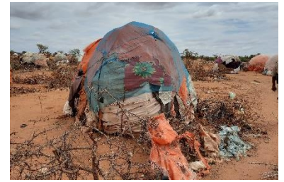
Plastic sheeting solutions are not very durable in the Somali climatic context. Buul in Doolow, Jubaland – CC Enrique Sevillano Gutiérrez, CRAterre
