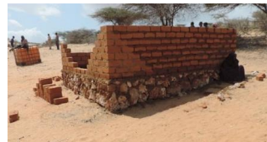
Elevation of CSEB walls - © IOM
