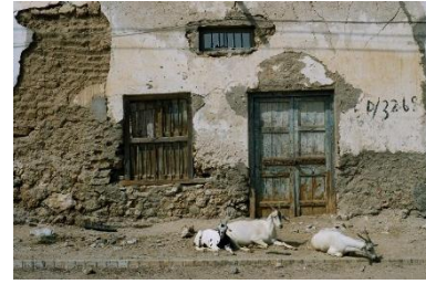
Adobe is usually not visible in urban houses, where it is protected with a plaster. Here, because of a lack of maintenance, we can clearly see an adobe wall in Berbera, Somaliland – CC Tristram Sparks
