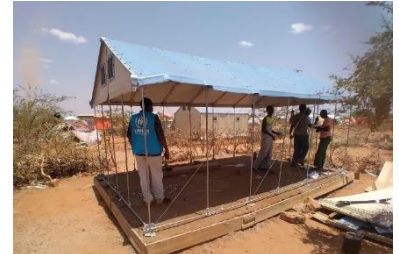
Refugee housing unit under construction in Doolow, Jubaland – © UNHCR
