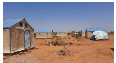
Refugee housing units in Doolow, Jubaland – © UNHCR
