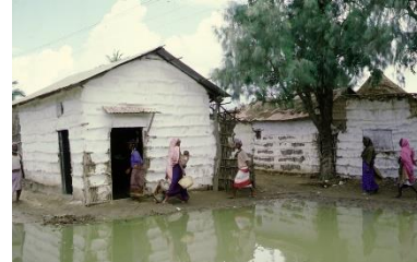
These baraako houses are built on a small earth mound what helps protect them from common flooding. Janaale, South West State © Thierry Joffroy, CRAterre
