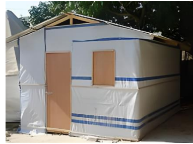
Emergency shelter built with timber and plastic sheet with CGI roof – © Shelter Cluster Somalia
