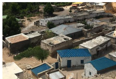
Mix of flat and sloped roofs in Eyl, Puntland – CC Heimo Liendl
