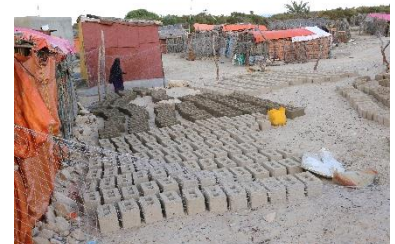
Production of cement hollow blocks in Puntland – CC Heimo Liendl
