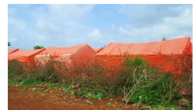
Shelters built with Emergency Shelter Kits (ESK) in Baidoa, South West State – CC Enrique Sevillano Gutiérrez, CRAterre
