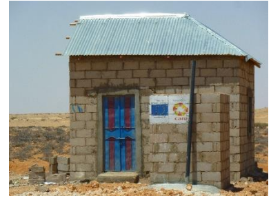
Shelter built with cement blocks with possibility of extension in Garowe, Puntland – CC Malini Morzaria / EU-ECHO
