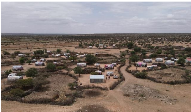
Village of Caramadaw (Somaliland), where each compound has a clear limit with the courtyard fence, a courtyard with shadowed exterior spaces, and different constructions for different uses – CC – UNDP - Said Fadhaye
