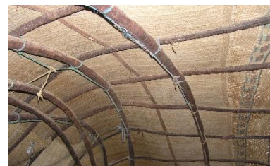
Aqal structures can last for more than 10 years when the elements are well selected, treated and maintained – CC Shafi
