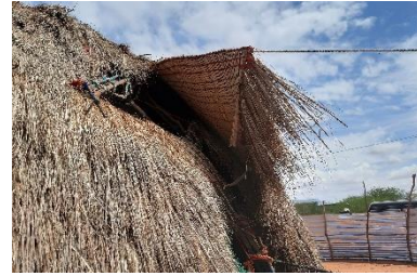
Aqal have simple mechanisms for the control of inner ventilation and temperature. Aqal in Doolow, Jubaland – CC Enrique Sevillano Gutiérrez, CRAterre
