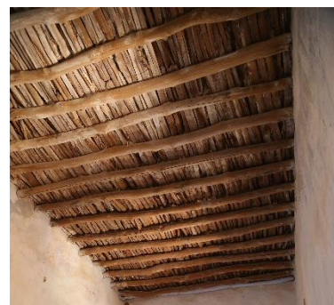
Flat roof built with timber in Eyl, Puntland – CC Heimo Liendl
