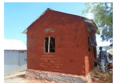
Finalized CSEB shelter in Kismaayo, Jubaland – © Shelter Cluster Somalia
