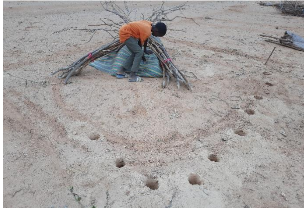
Holes made for the poles of aqal in Doolow, Jubaland – CC Enrique Sevillano Gutiérrez, CRAterre
