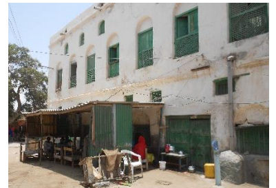
Whitewashed stone building with windows with wooden lattice to provide shading and privacy inside the houses. Small cafe with veranda, spaces with a lot of use during hot conditions. Berbera, Puntland – CC Ignacio Gallego
