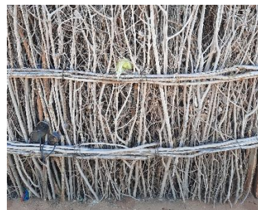
Wall of an unplastered baraako in Doolow, Jubaland – CC Enrique Sevillano Gutiérrez, CRAterre
