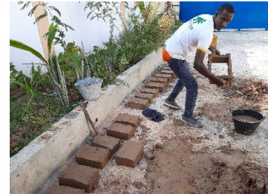
Adobe (sun-dried earth bricks) are a potential locally produced alternative to the traditional wattle and daub technique which can have a negative impact in deforestation – CC Enrique Sevillano Gutiérrez, CRAterre
