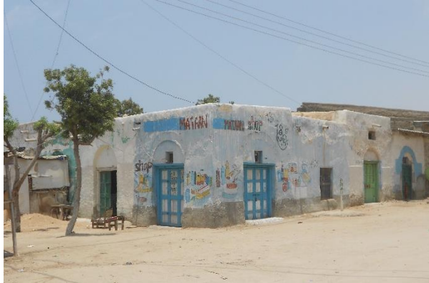
Masonry construction (adobe and/or stone, as they are not visible with the plaster) in Berbera, Puntland – CC - Ignacio Gallego
