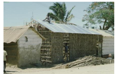
Baraako under construction in Jenaale, South West State - © Thierry Joffroy - CRAterre
