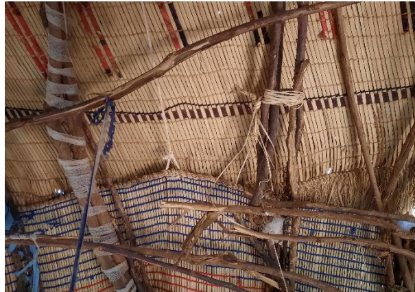
Detail of mats and structure in an aqal in Doolow, Jubaland – CC Enrique Sevillano Gutiérrez, CRAterre
