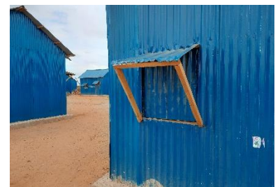
Shading devices help protect openings from solar radiation. Doolow, Jubaland – CC Enrique Sevillano Gutiérrez, CRAterre
