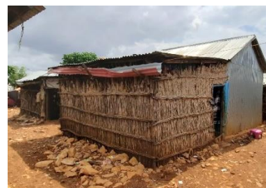
Extension of a CGI house using local materials and techniques ( baraako ). Baidoa, South West State – CC Enrique Sevillano Gutiérrez, CRAterre
