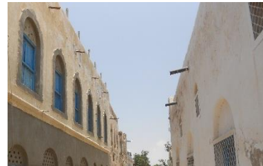
Flat roofs with tubes for the evacuation of rainwater. Berbera, Somaliland - CC Ignacio Gallego
