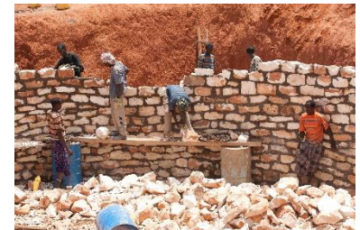
Construction of a rainwater catchment in Garoowe, Puntland - CC ICRC
