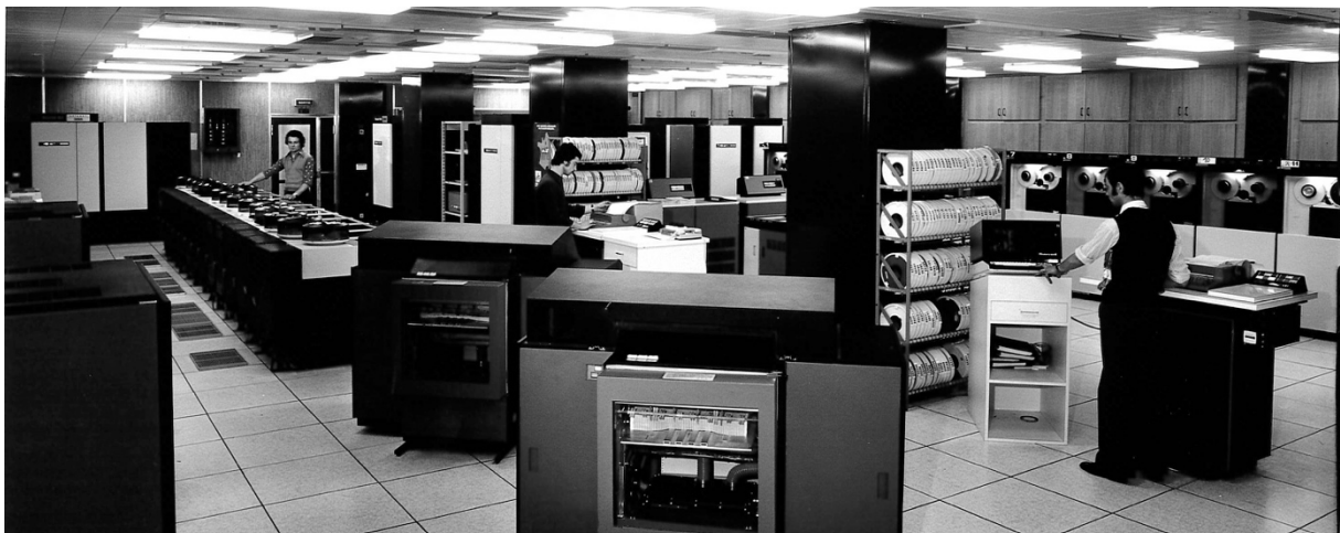
Figure 2. A powerful GE600 computer installed at Electricité de France (EDF) in the late 1960s.
