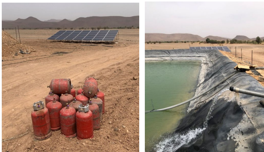
Figure 2. A water storage basin and solar panels in Mird; the latter are used (sometimes in combination with LPG) to pump up groundwater.
