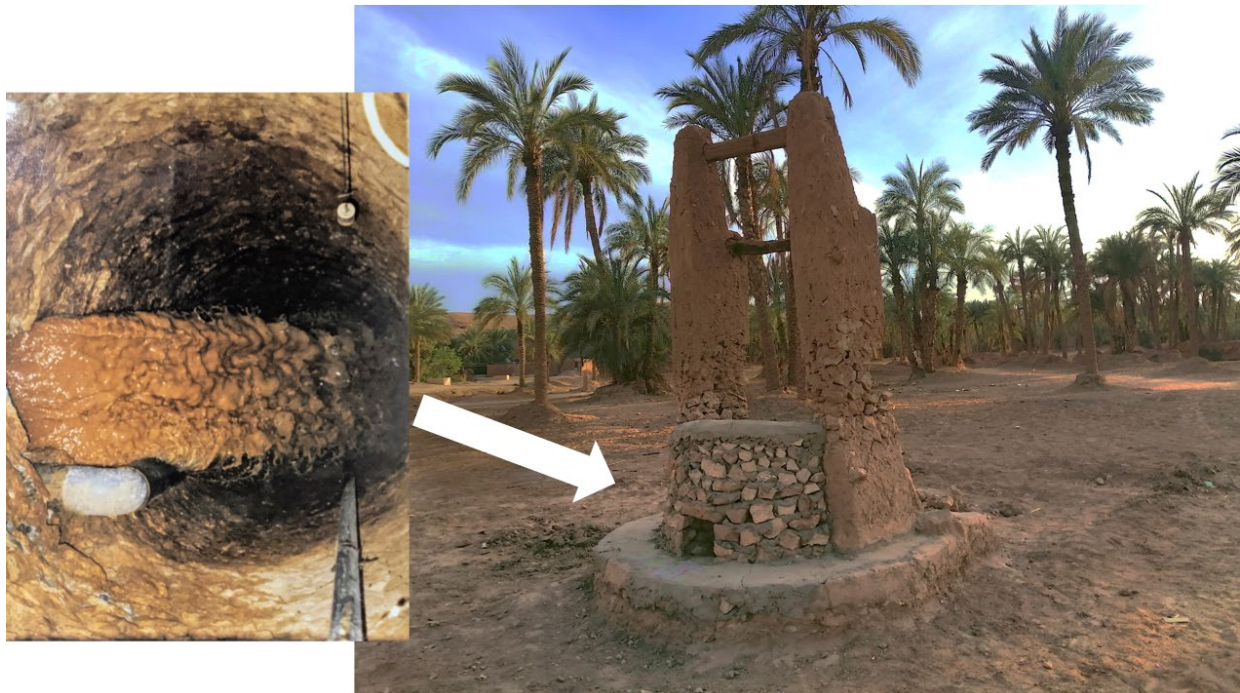
Figure 4. A recharge well, locally called abar baluàa (lit. swallowing well) in the oasis of Beni Isguen.
