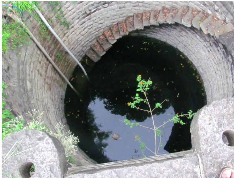
Figure 6. A typical large-diameter dug well in Randullabad that was constructed in the 1960s and 1970s.
