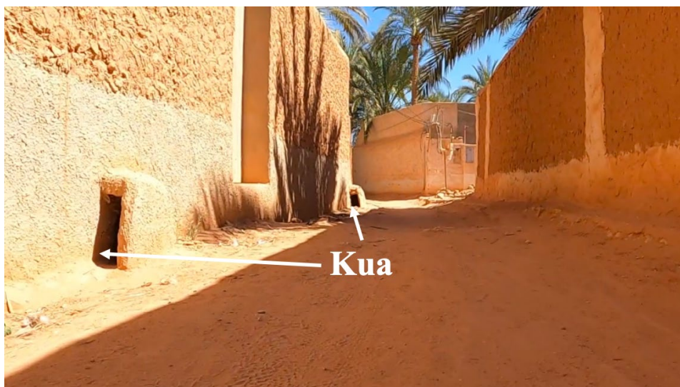
Figure 3. Intakes ( kua ) to gardens in the oasis of Beni Isguen.
