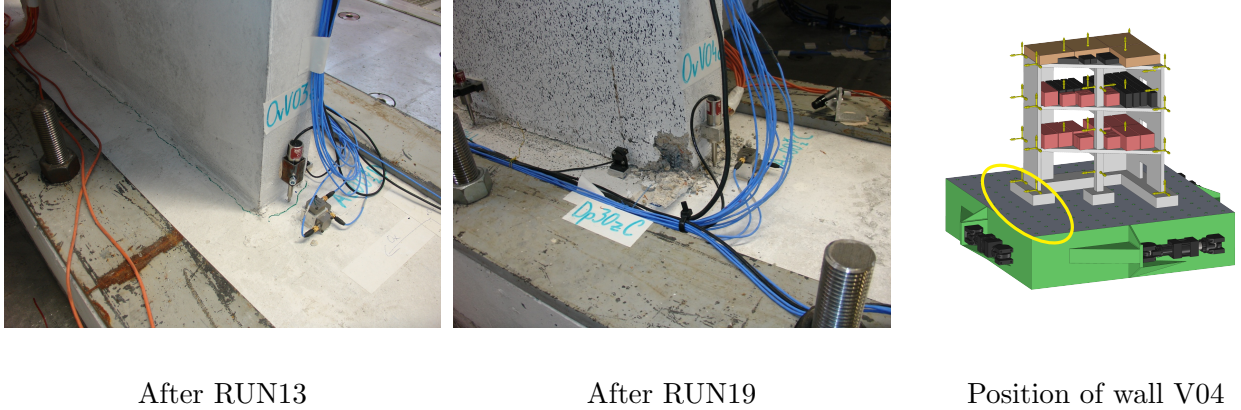
FIGURE 20: Main damage area of the SMART2013 specimen: base of the wall V04. (After RUN13) first crack appearing near the junction between wall and soleplate – sudden rupture of one or more vertical reinforcements. (After RUN19) rupture of the rest of the vertical reinforcements at the base of wall V04 – complete loss of rigidity between wall and soleplate (breathable crack) – high damage level to concrete.
