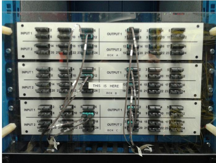
Figure 9.19: Dual  $12 \times 12$  fibre ribbon remapping modules in a 2U enclosure installed in a standard LHC rack in Point-5. 8 such dual modules will be required on ATLAS.
