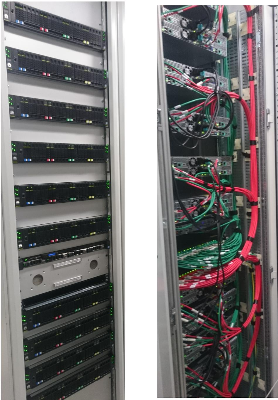
Figure 16.8: Photographs of a typical event processing rack configuration in [SDX1](#). The left photograph shows the front side of the servers, while right one the rear network interconnections to the rack-level switches.
