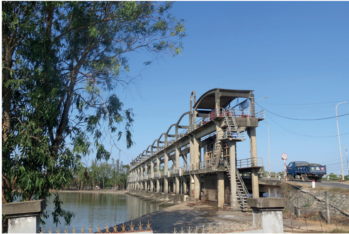
[ Figure 11.12 ] Dam sluice gate on the Ba Lai River to block saltwater intrusion
