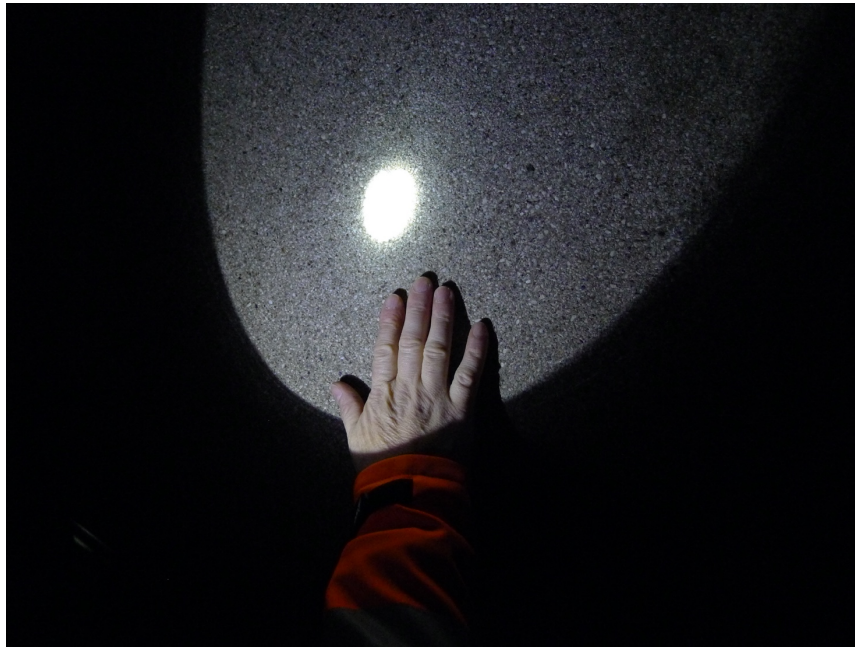
Figure 1. Inspecting a water reservoir: touching (© J. Denis)
