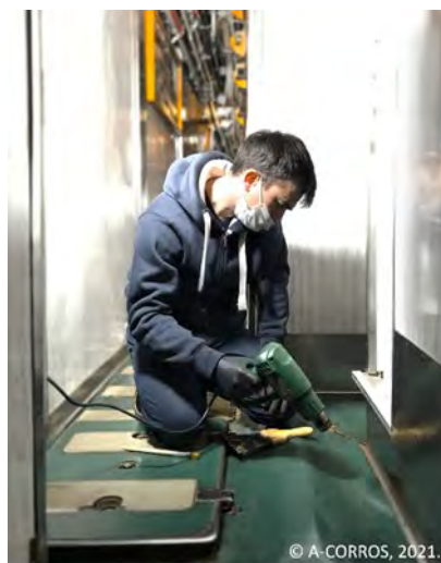
Figure 16. Zone de restauration test du PVC, ©A-CORROS 2021.
