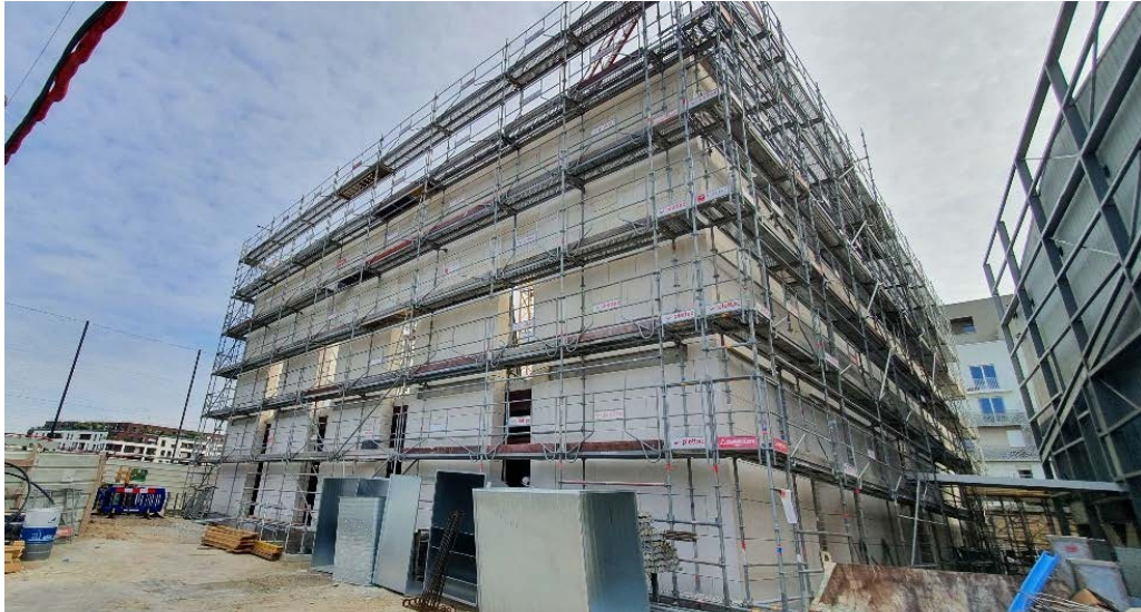
Figure 2: Gymnase Alain Mimoun – Artibal Architectes – Issy les Moulineaux – 2022
