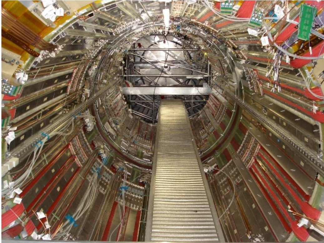
Figure 17.7: Access platform inside the inner warm vessel during ID construction.
