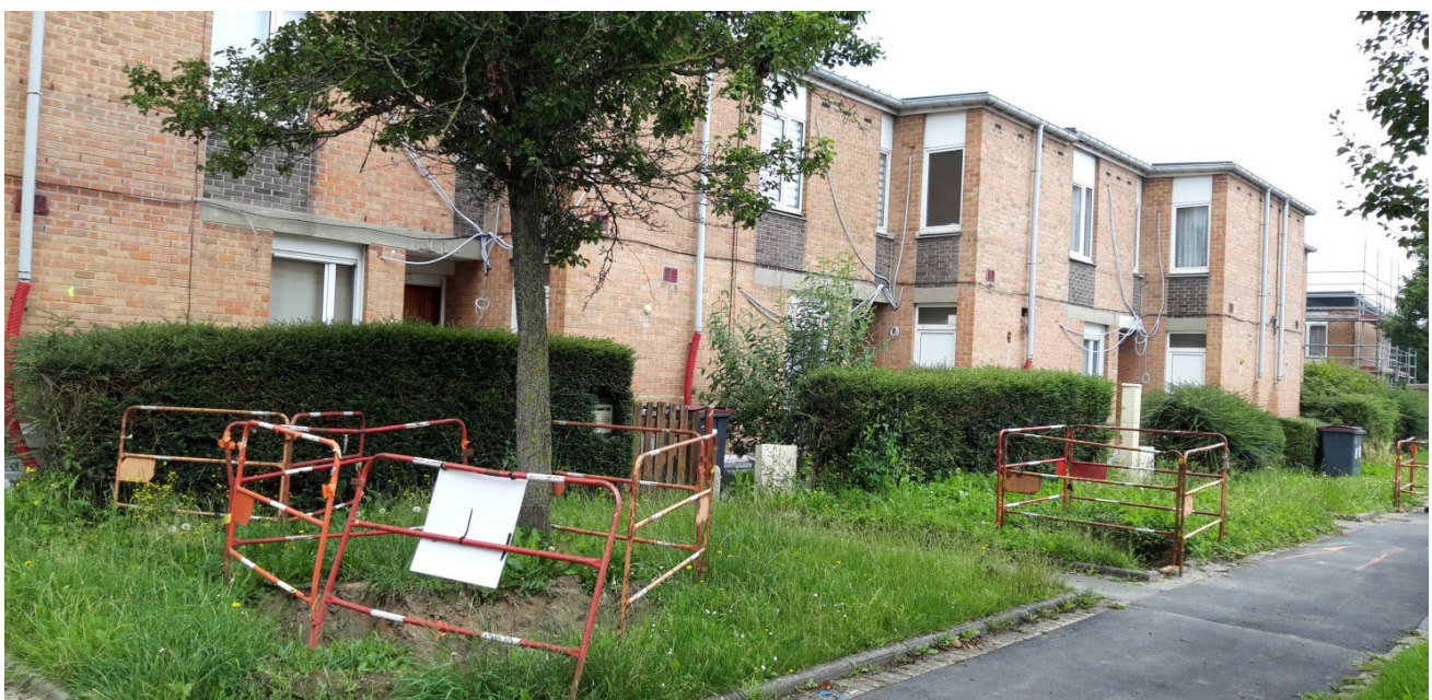
Figure 4. Public space affected by energy network upgrade in Wattrelos.
