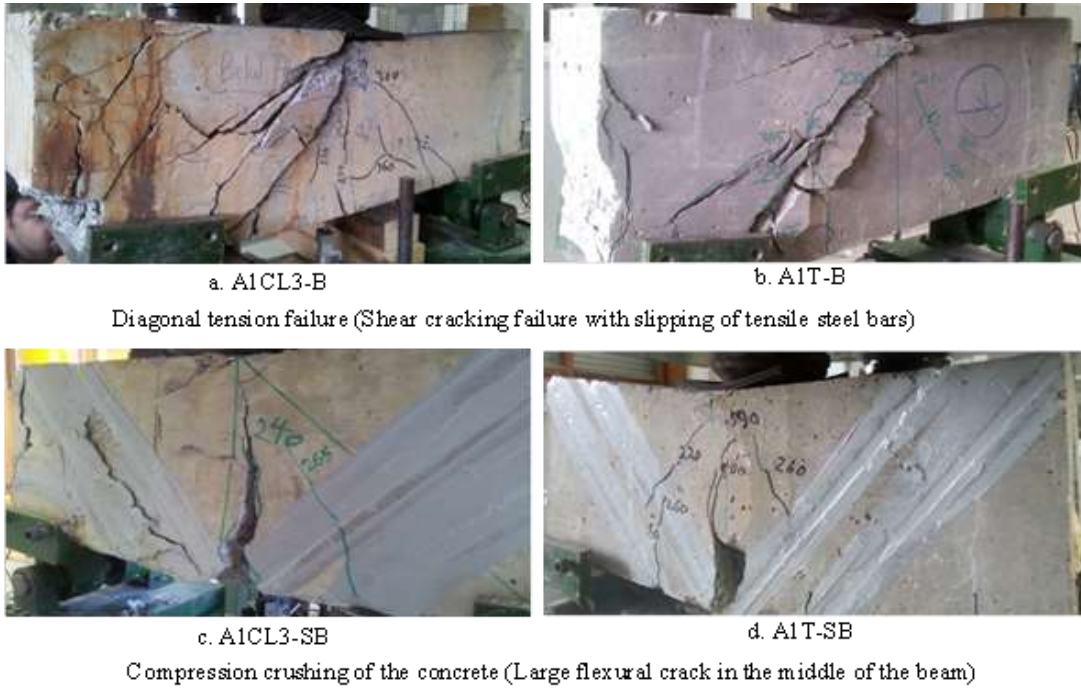
Figure 6 Experimental modes of failure for all tested beams
