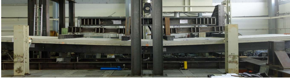
Figure 15: Photo of the specimen BM-1 after the test.
