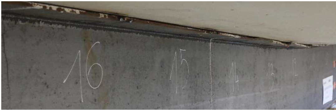
260 Figure 16: Plastic buckling of the upper flanges of the U-shaped steel profile at locations of shear connectors.
