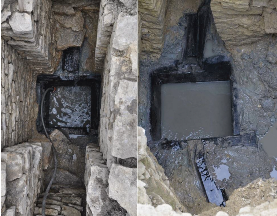
Figure 4. THE MANHOLES OF THE «COMMODIAN» NETWORK AND THE WOODEN SETTLING BASINS (O. DE CAZANOVE) (ON THE LEFT, 3000 BASIN = 1,08 \times 0,66 \times 0,44 M / ON THE RIGHT, 3350 BASIN = 1,08 \times 0,81 \times 0,46 M)
