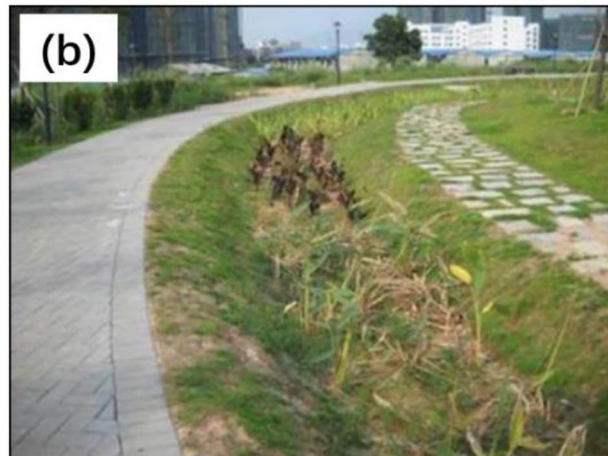
Fig. 9 Xincheng Park in the Guangming District of Shenzhen, Guangdong province: a site layout after renovation, and b a grass swale in the park. Image also shows permeable pavements alongside the grass swale
