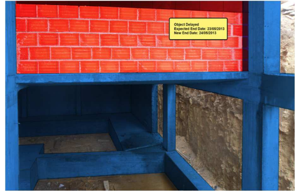
Figure 5: (left) 3D KMS for virtual rendering of greening on building's roofs [91], (right) a tag note assigned to a delayed wall using AR mobile handheld [93].
