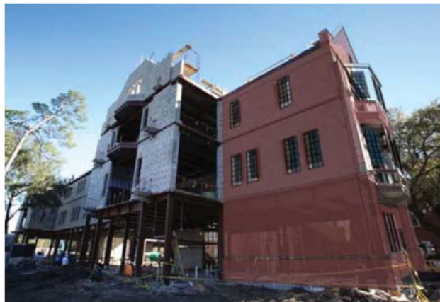
Figure 6: Superimposed 3D BIM model over worksite construction progress documentation using AR mobile handheld [96].
