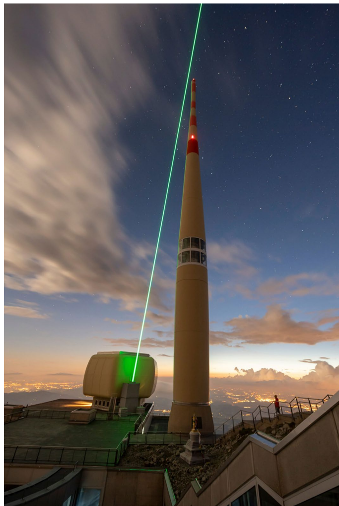
Fig. 1 | Image of the 124-m-high telecommunication tower of Säntis (Switzerland). Also shown is the path of the laser recorded with its second harmonic at 515 nm.
