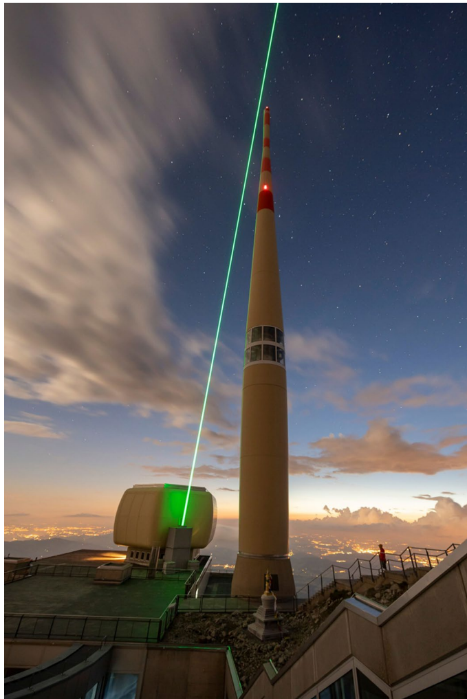
Fig. 1 | Image of the 124-m-high telecommunication tower of Säntis (Switzerland). Also shown is the path of the laser recorded with its second harmonic at 515 nm.
