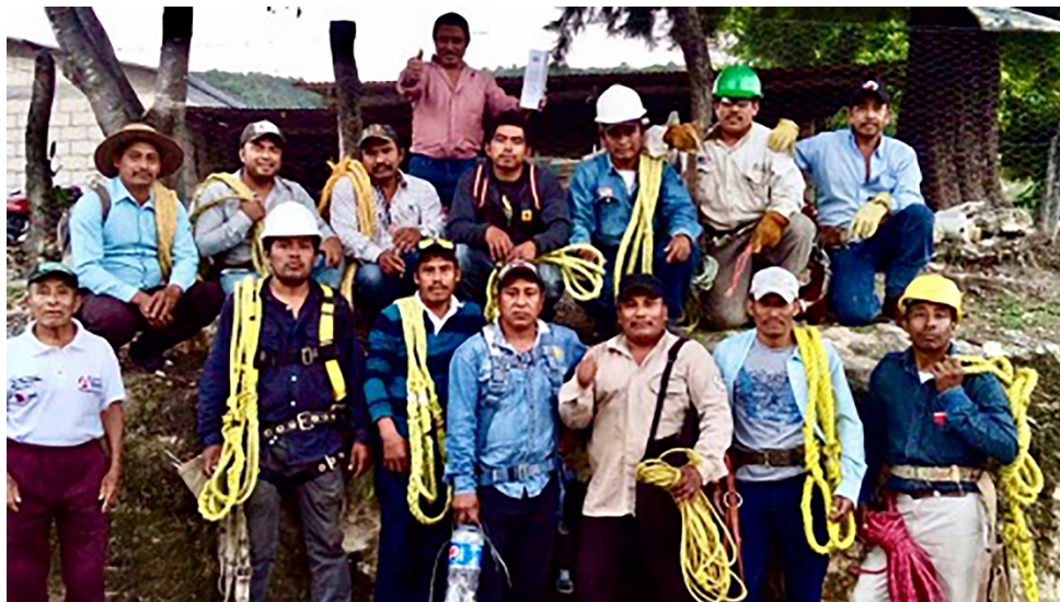
Picture 4. A group of electricians of Luz y Fuerza del Pueblo after performing an intervention on the electrical grid. Zapaluta region, November 2019. Source: LyFdp.
