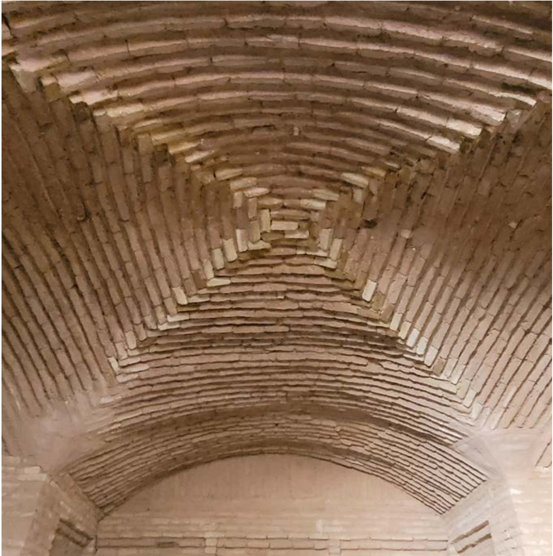
A Four-Arch Vault. Using Brick instead of Adobe in the Intersection of Ridges. Khaje Khezr. Yazd
