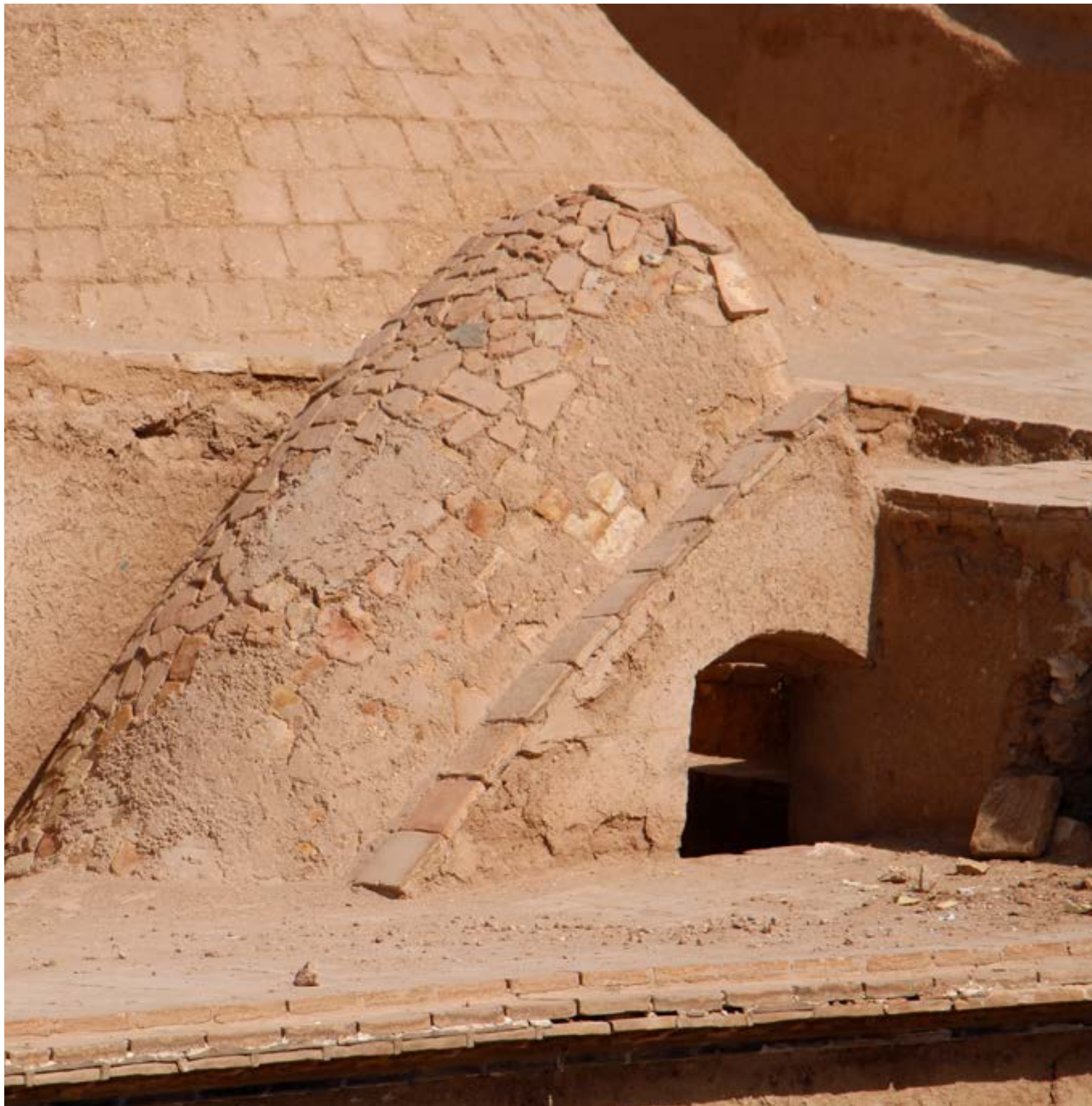
Roof Access. Falsafi House. Naghib-ol Ashraf Alley. Yazd
