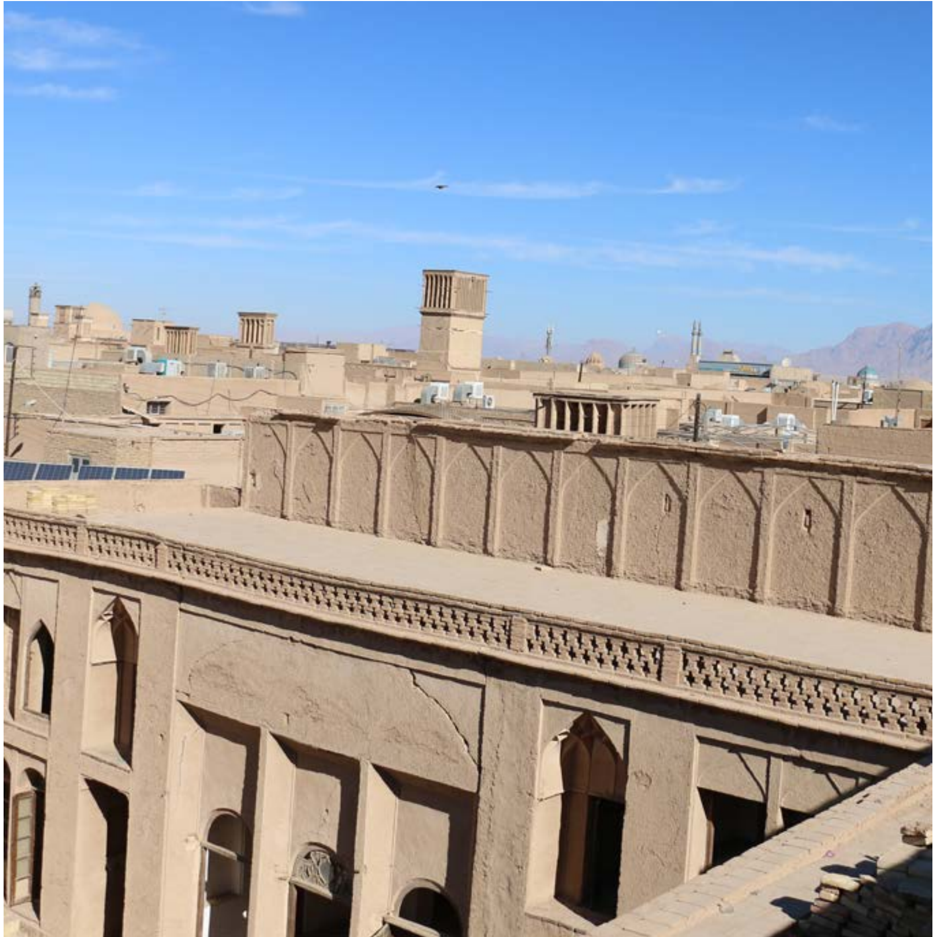
Brick Parapet Wall. Ostovar House. Golchinan. Yazd
