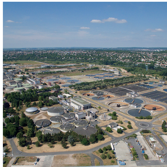
Europe's largest wastewater facility, the Seine-Aval plant at Achères, near the Seine-Oise confluence. Photo: SIAAP Emmanuel RICHE ODYSSEE_V360 Mrs ZZ, with permission
