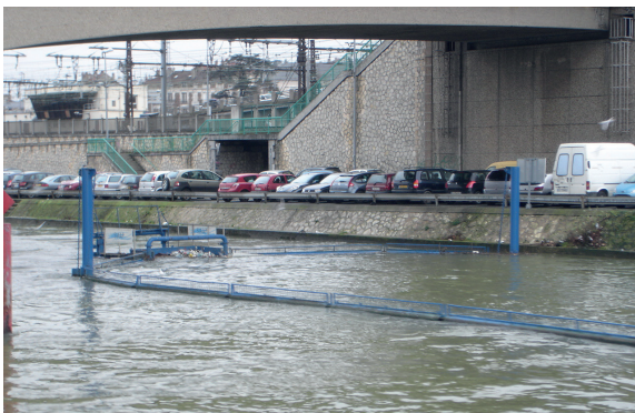
Typical urban river bank devoted to car traffic. Floating debris captured by the sewage treatment institution. Photo: Laurence Lestel
