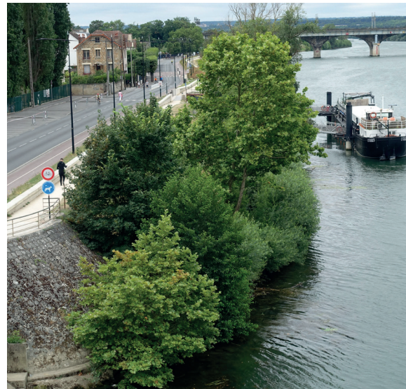
Typical river rehabilitation, with wooded slope and pedestrian walkway (Seine at Sartrouville). Photo: Laurence Lestel
