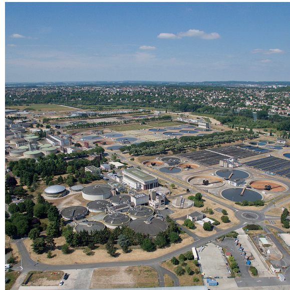
Europe's largest wastewater facility, the Seine-Aval plant at Achères, near the Seine-Oise confluence. Photo: SIAAP Emmanuel RICHE ODYSSEE_V360 Mrs ZZ, with permission
