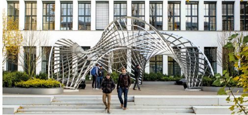
(b) An example of asymptotic gridshell (picture :[10])
