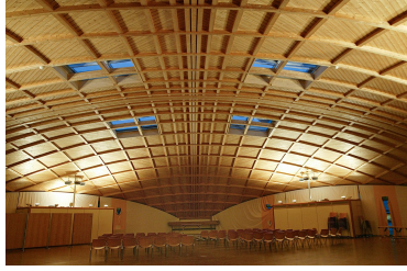
(a) EPFL Polydome: an example of geodesic gridshell (picture : EPFL-MEDIACOM, distributed under Creative Commons 4.0 License.)
