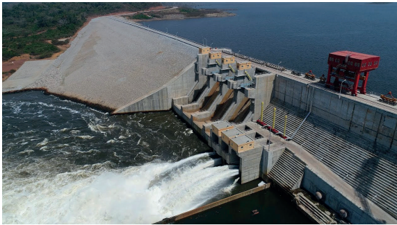
Nachtigal Dam. Photo: World Bank, with permission
