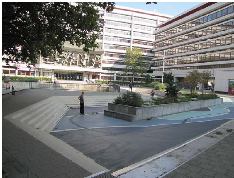
Figure 4: Bentheplein water square in Rotterdam created in 2013 for the rainwater management
