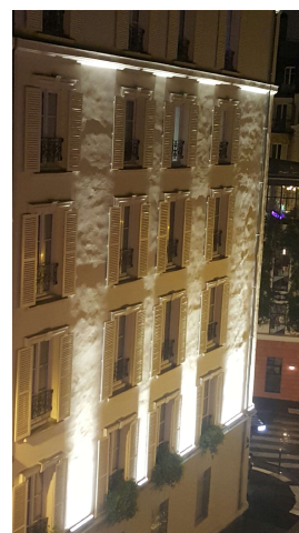
Figure 1. The planarity defects of the facade are highlighted by a grazing lighting, which is the basic principle of RTI.
