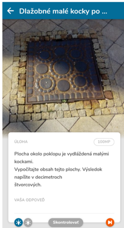
Figure 4 Small paving tiles
