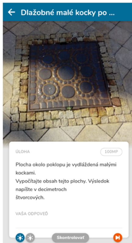
Figure 4 Small paving tiles
