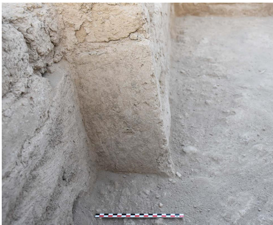
Fig. 11 – plaster of the redan of wall 3088, from the south.
