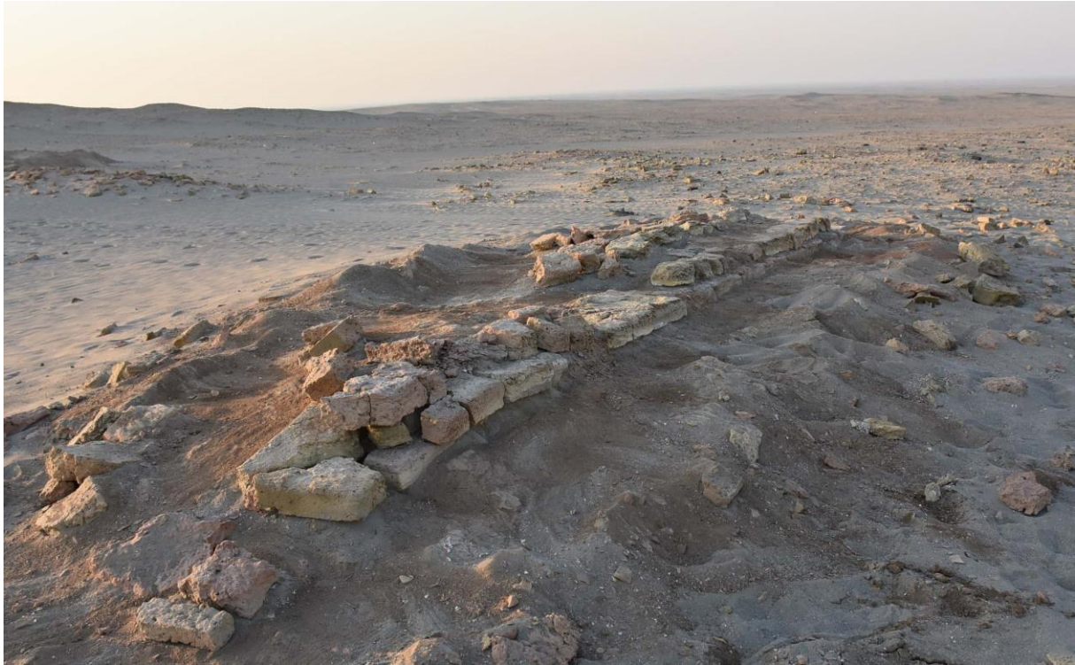
Fig. 15 – The baked brick facing of the northern facade of temple B50, from the northeast.
