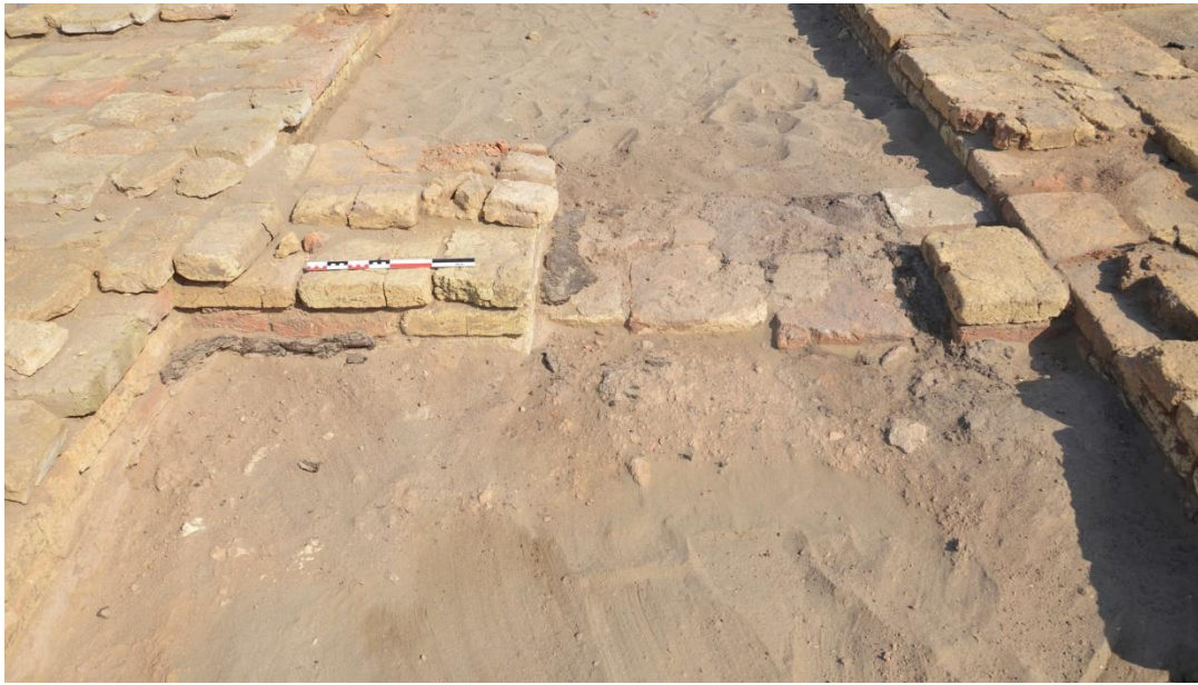
Fig. 9 – Preserved part of room 1617, showing remains of a bitumen floor, from the west.
