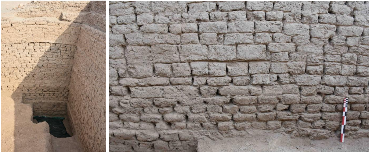
Fig. 6 – Left: Southeast and Northeast walls of room 3019 being cleared Right: Detail of the masonry of the southeast wall.
