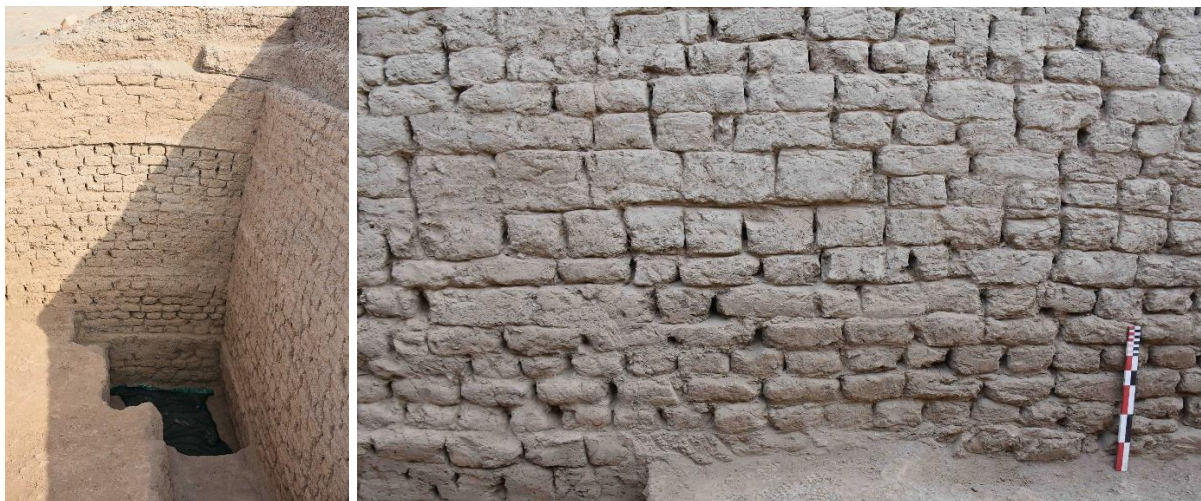
Fig. 6 – Left: Southeast and Northeast walls of room 3019 being cleared Right: Detail of the masonry of the southeast wall.
