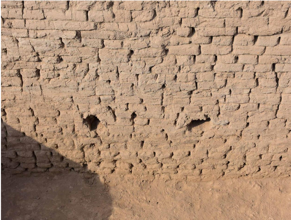
Fig. 8 – Anchor points in the northwestern wall of Room 3019.
