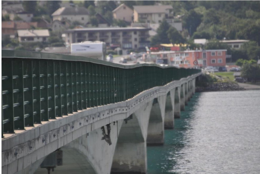
Figure 1 View of the Savines bridge. The hinges allow large deflections that are visible at each mid-span (photo credited to J.M. Torrenti)
