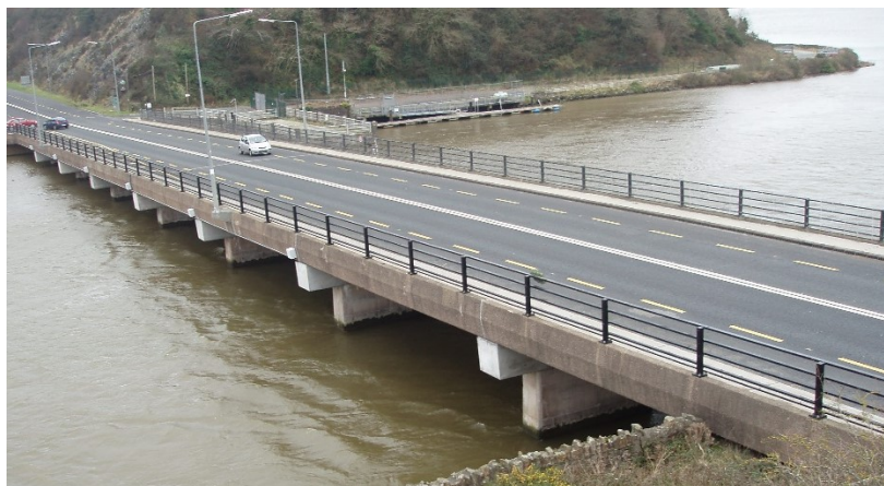
Fig. 6. Ferrycarrig Bridge showing the seven repaired crosshead beams.
