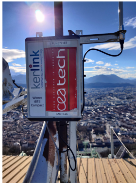
Fig. 3. Gateway installed on the roof of the cable-car arrival station at Bastille, overhanging the city of Grenoble, France.
