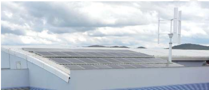
Fig. 2: Photovoltaic panels and vertical axis turbine in the HRGS.
