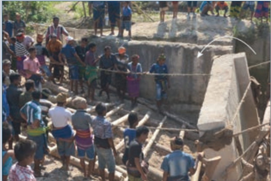
Capstone extraction, first movements of pull and positioning gently on the wood ramp
