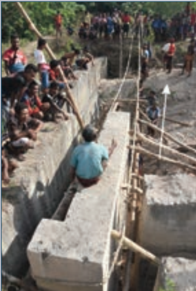
Capstone extraction, first movements of pull and positioning gently on the wood ramp
