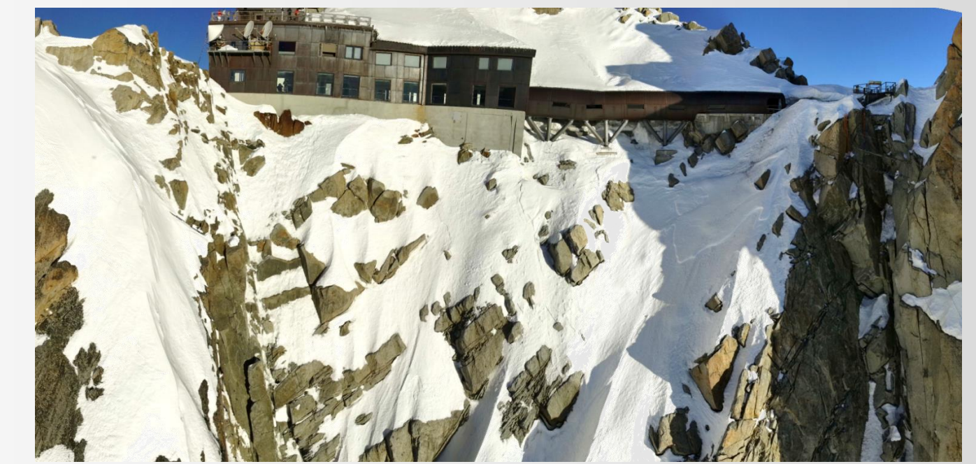
Figure 3B: SE face of Aiguille du Midi with substantial snow cover.
