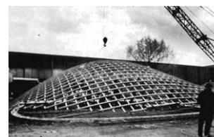
Figure 7: Construction of the Essen Gridshell [ibid].
