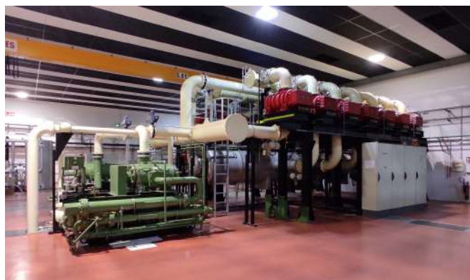
Fig 3. Wind tunnel MARHy pumping group
