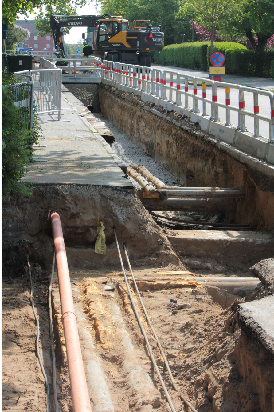
Figure 13 Picture taken of the pipes and cables in the subsurface during the excavation at Trastvägen (Lund). The photo shows several central heating distribution pipes, electrical, internet and telephone cables.
